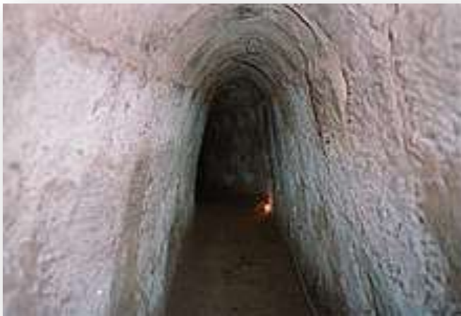
Part of the tunnel complex at Củ Chi, this tunnel has been made wider and taller to accommodate tourists.
